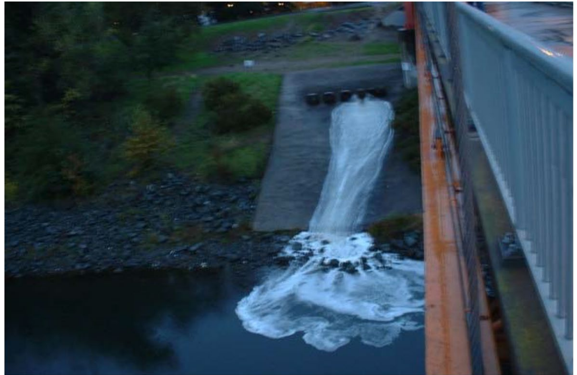
Storm Drain Discharges into American River
