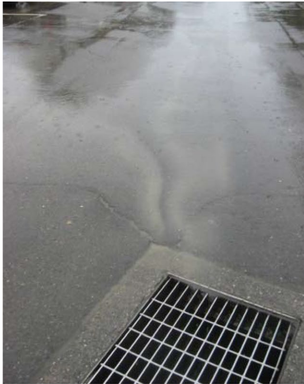
Drain Inlet - Campus
