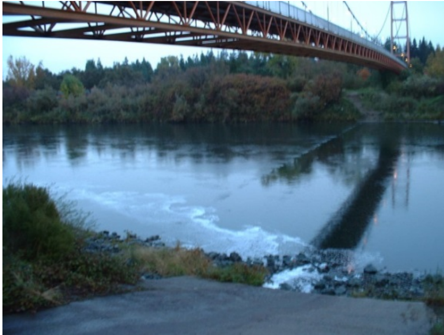
Outfall – Guy West Bridge
