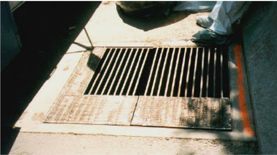
FIGURE 2 Modified drain inlet.
